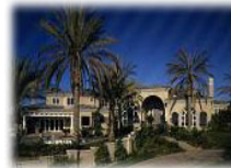
1st Place— National Builders 1989
